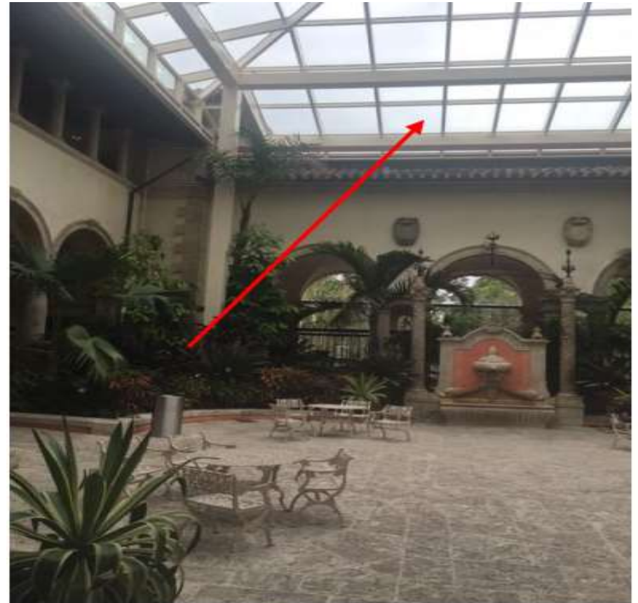
The high-impact glass canopy/skylight covering Vizcaya's Courtyard protects its culturally and historically significant collections. Photo by: Bonnie Hanchett
