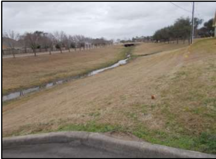
Lone Tree Creek Channel near StockBauer Drive after the 2005 expansion project. Photo by: Joyce Price/FEMA
