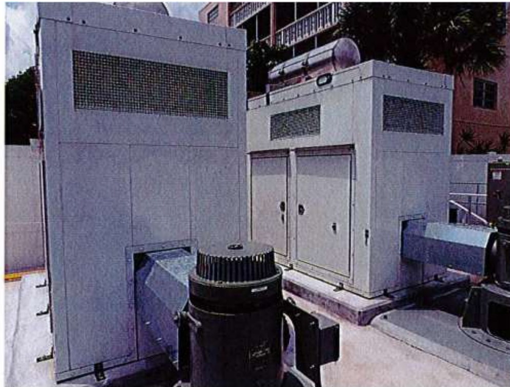
Pump station withdraws storm water from culvert and discharges to wells. Photo courtesy of Florida Division of Emergency Management
