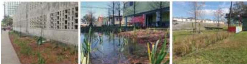
1. to H. A bioswale along Pipeline St., a NOAA bio-retention cell, a bioswale near N. Broad St.
