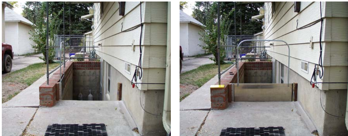
This house in Fort Collins, Colorado, was faced with basement flooding. The stairwell's retaining wall was raised and a removable closure fits in grooves in the walls. This project relies on human intervention – if someone does not slide the board in place, the building will not be protected.
