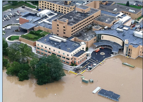
Figure 4-6 Aerial view showing effective protection of Lourdes Hospital from flooding as a result of Tropical Storm Lee
