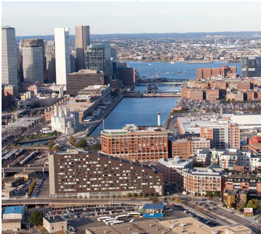
The Fort Point Channel is a major inundation point for the 1 percent annual chance flood risk in the year 2070. Photo: Landslides Aerial Photography / Alex MacLean
