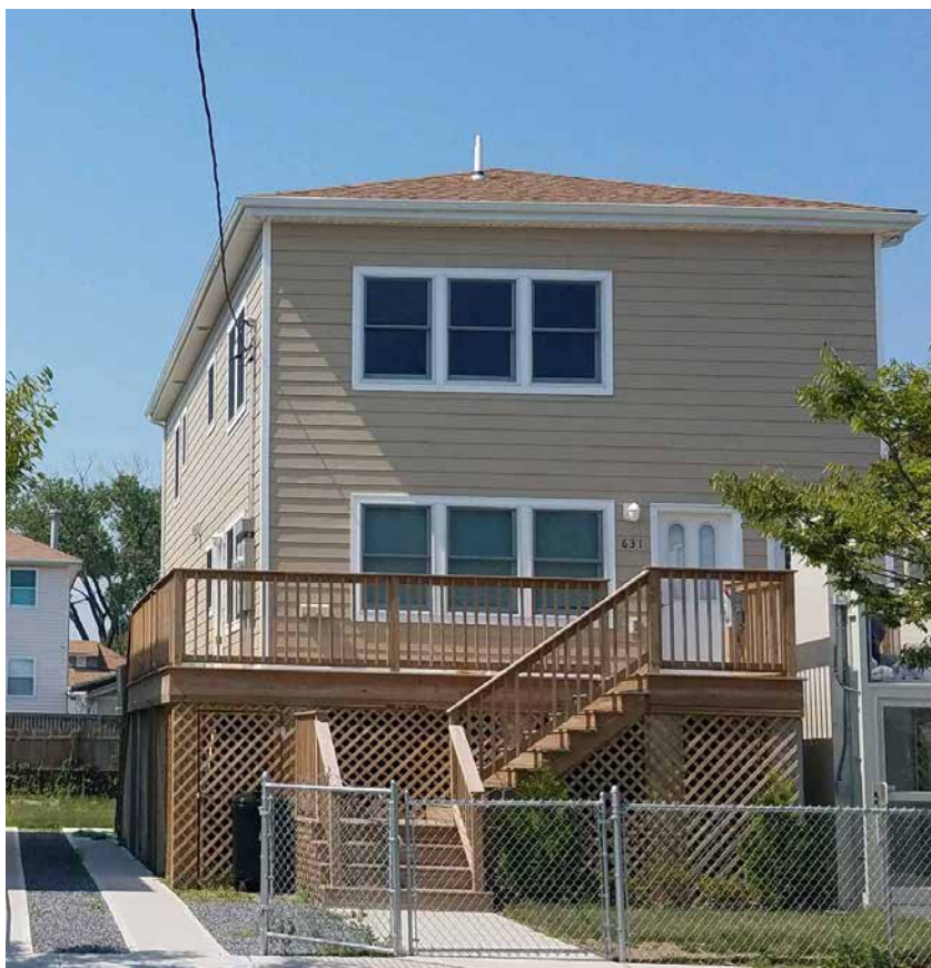
Elevated home in the Arverne neighborhood of Queens, New York. Photo source: NYC Housing Recovery Operations
