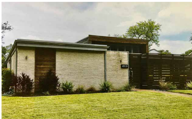
House in Meyerland, Houston before elevating.
