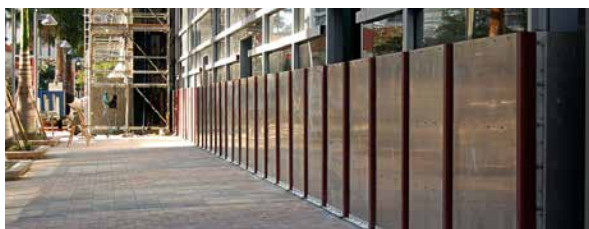
Flood panels connected to removable posts. Photo: Flood Panels LLC
